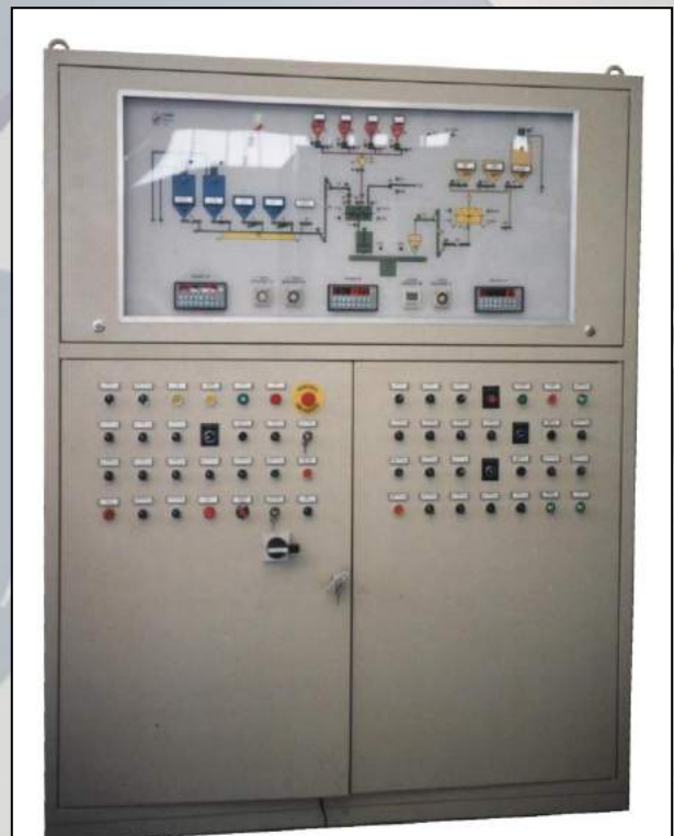
Q.E. con sinottico e comandi manuali da selettore. Electric board with synoptic and manual controls from the selector.
