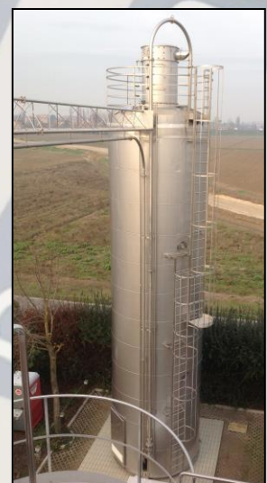
Silos in AISI304. Stainless steel storage bins.
